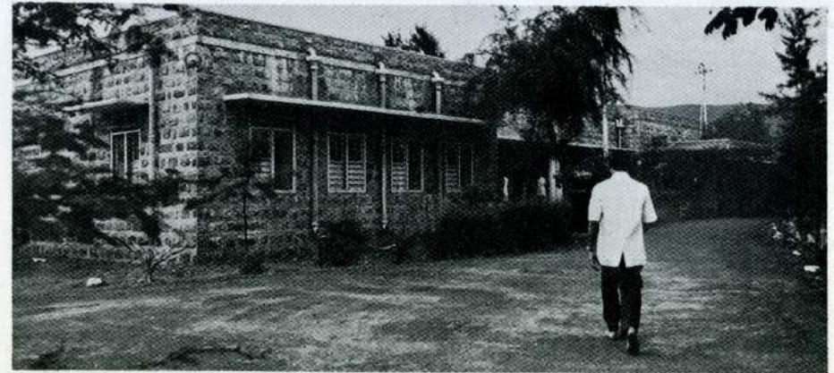
The T.B. Hospital. The Caltex Refinery is a major donor to this hospital, started 10 years ago. The X-ray equipment was presented by our Refinery.
