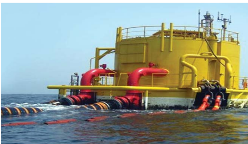
Single Point Mooring Project (SPM), Visakh Refinery.
