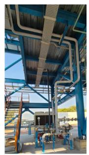
The in-house developed insulating coating for low temperature services is for mitigating condensation corrosion of assets and can be used upto temperature of -20 deg. C.
