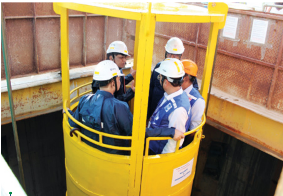
C&MD, HPCL in a review visit to HPCL LPG Cavern project at Mangalore, a testament to our commitment to safety and energy security
