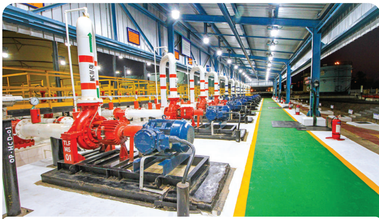
► VFDs for product pumps and LED lighting in sheds for energy conservation
