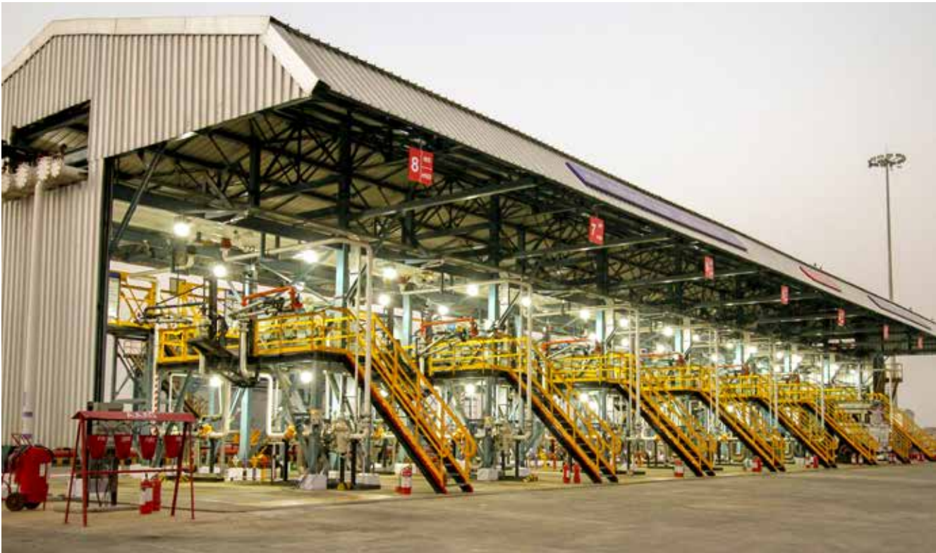
Flame proof LED lighting at tank truck loading gantry at one of our POL locations
